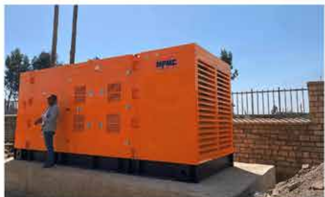
Kenya, Perkins, Construction
